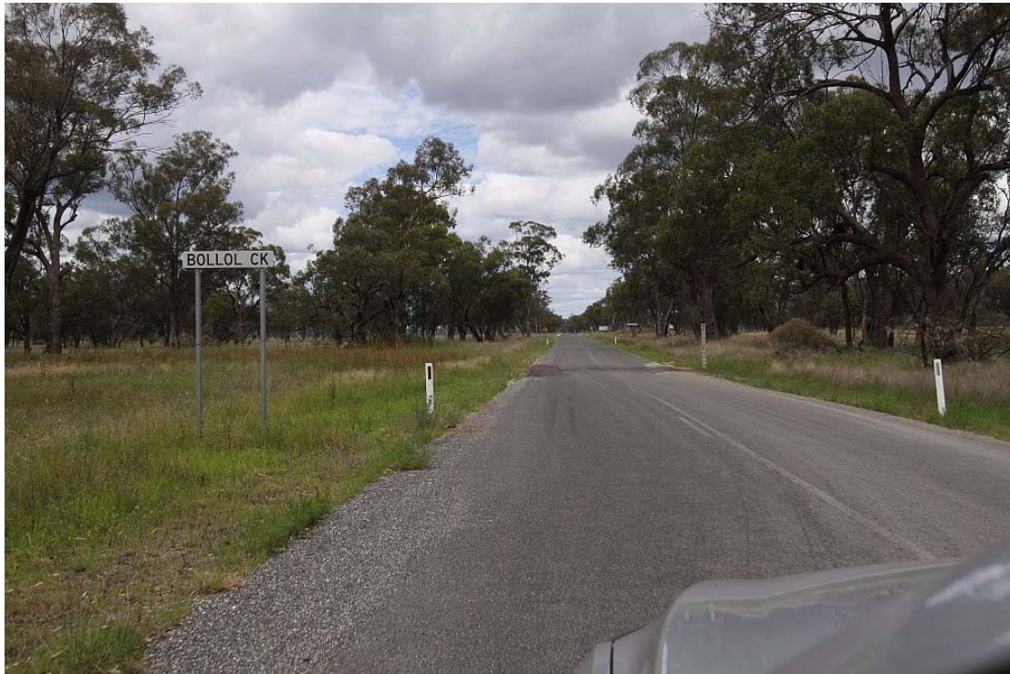
Photograph 5 – Ephemeral Bollo Creek Crossing
