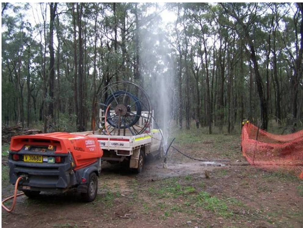
Photograph 2 – Airlift development of monitoring bore
